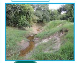
2-YR Level of Service (LOS) Rainfall event the stream is capable of containing within HCFCD right-of-way.
